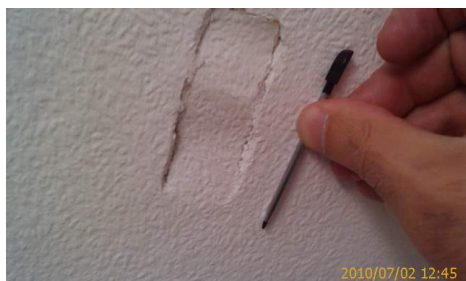
Stairs/ landing 2-Ceiling
